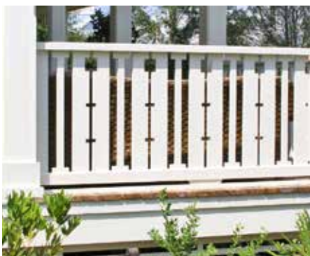
Builders may distinguish themselves with two to three styles of distinctive custom-cut board pickets
