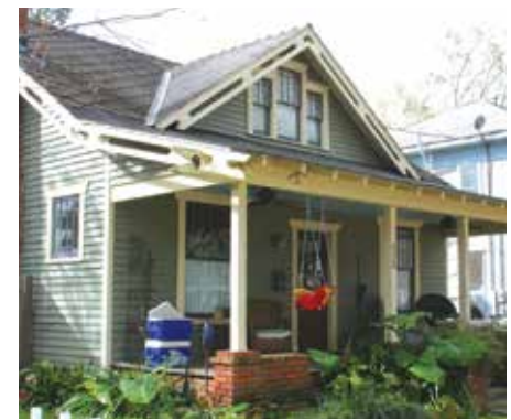
One and one-half-story side gable
