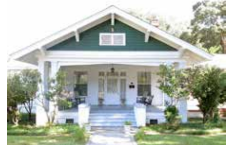
Front porch is integrated into the front gable main body mass
