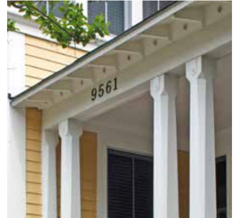
Square chamfered posts and railing with sawn balusters
