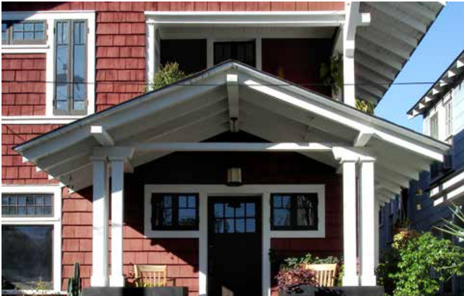
Wide fascia boards supported by robust brackets project from the front of this bungalow porch
