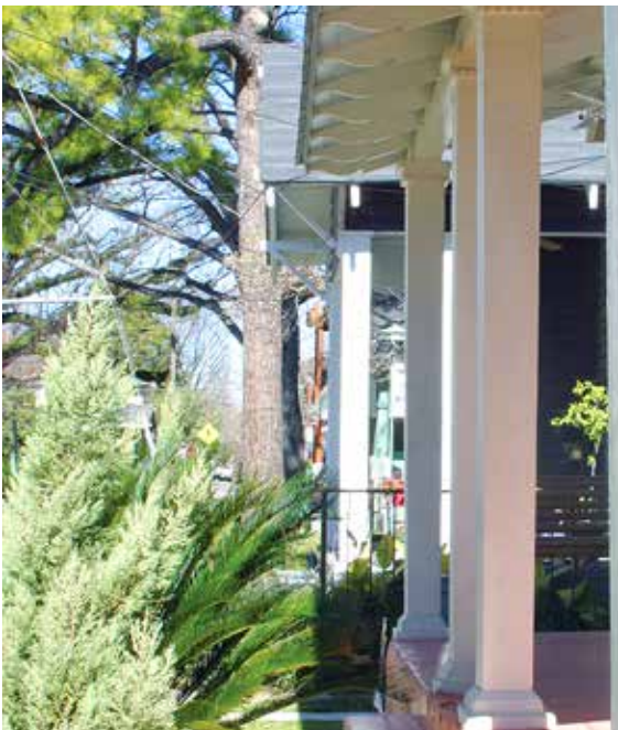
Porches that provide shade and outdoor living space
