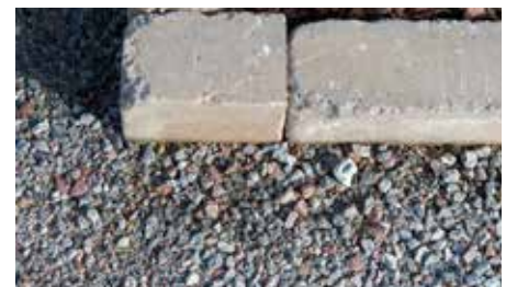
Stone aggregate driveway with concrete paver
