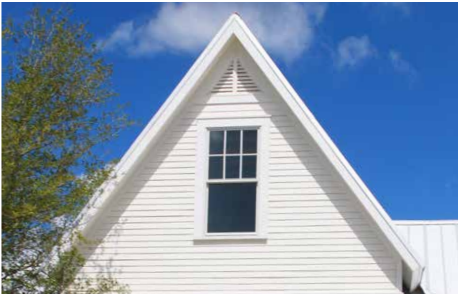
Sloped box eave with articulated gable vent
