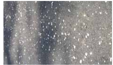
Asphalt driveway with seeded shell
