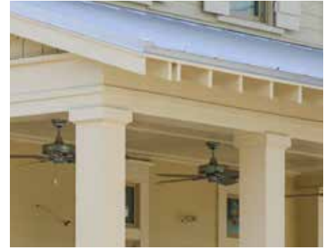
Exposed rafter tails
