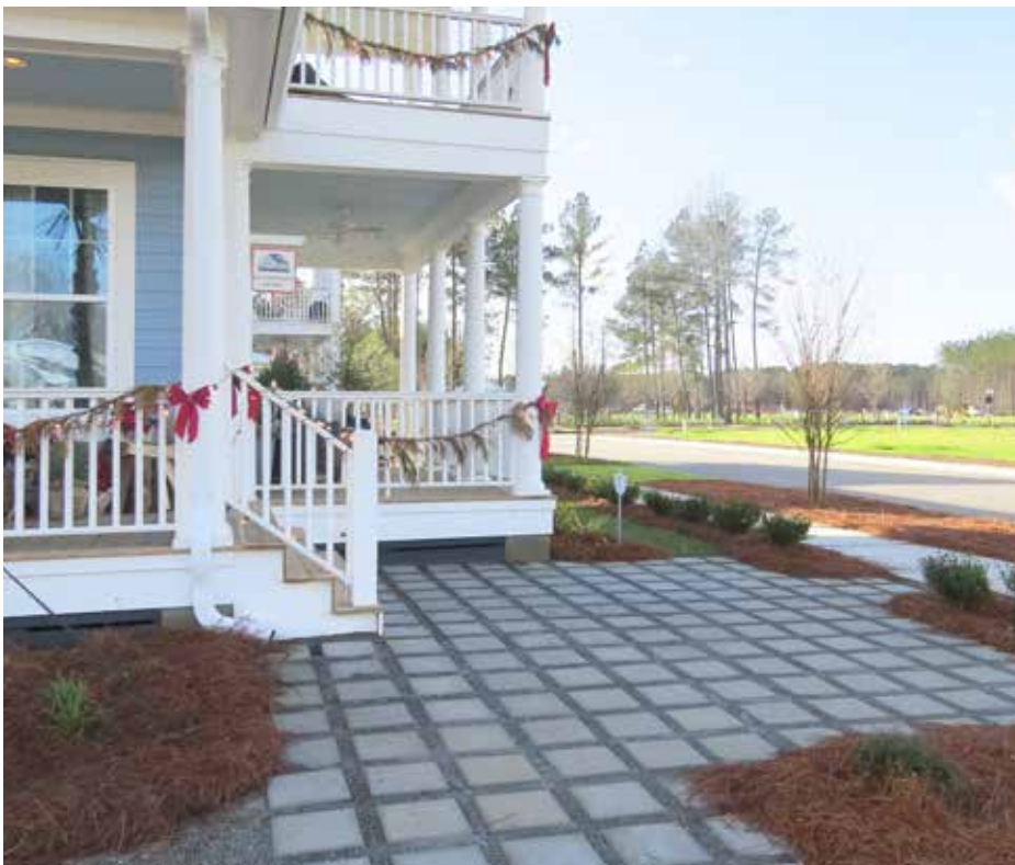
Stone aggregate/concrete paver walking path
