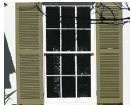
Operable windows and shutters
