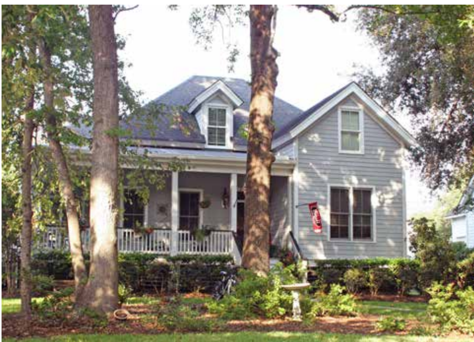
One and one-half-story Gable L massing with separate porch roof from Main Body
