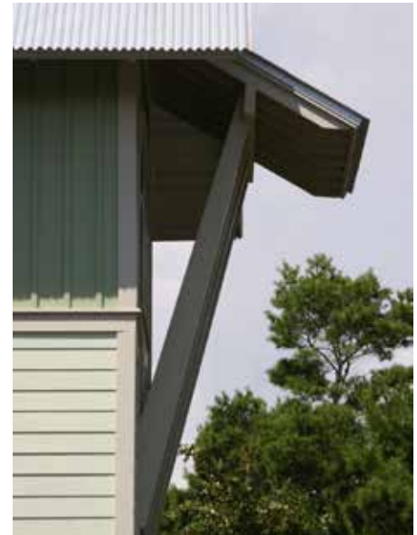
Rafter tails supported by brackets and cross beam
